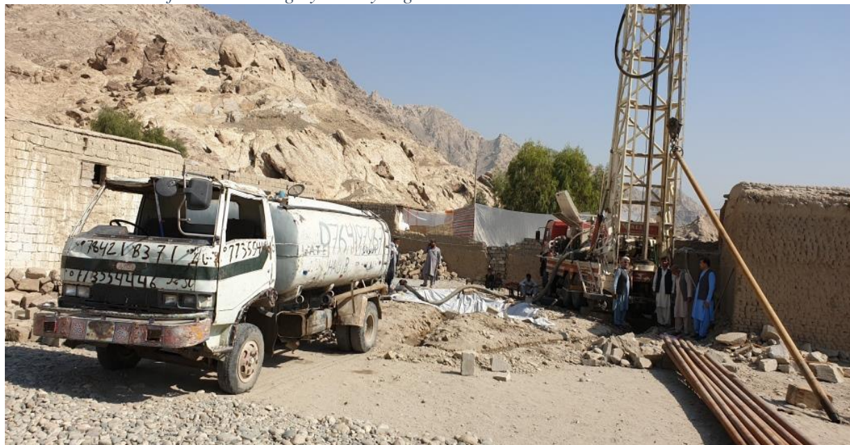
Photo 9: The view of a well drilling by Rotary Rig Machine in Daman
